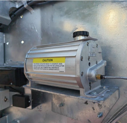
E-SERIES Electro-hydraulic brake (1,200 psi)
